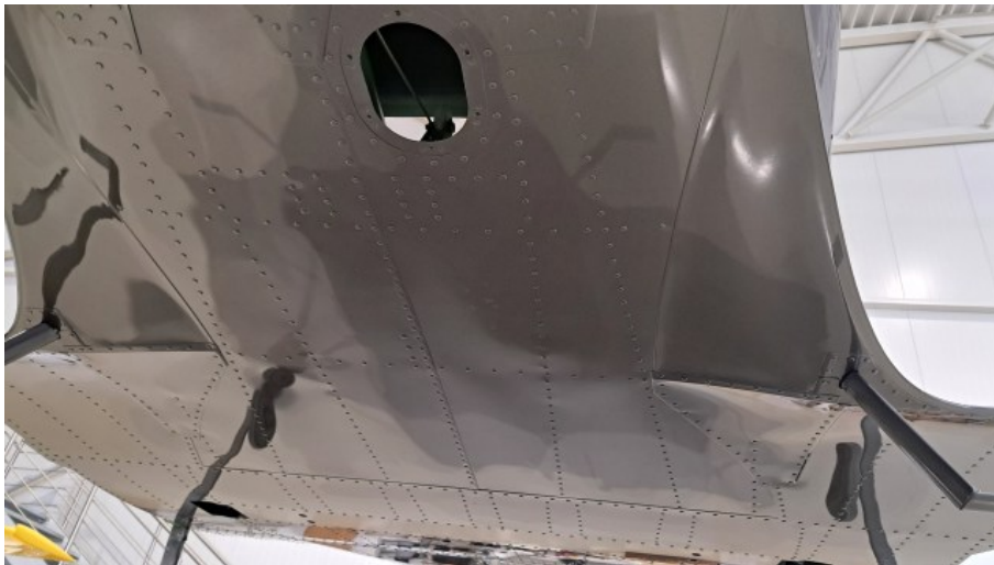
Fig. 6 Inspection hole on fuselage bottom through which the missing rivets can be installed. Installation involves some effort required to reach the rivet installation location.
