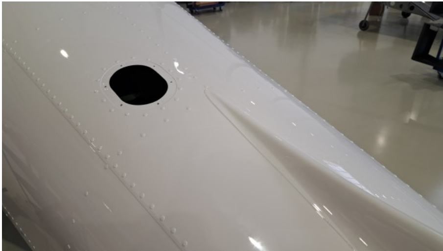
Fig. 1 Inspection hole (after removing the cap) on the upper side of the fuselage. Through this hole the internal structure of the fuselage can be visually inspected for missing rivets.
