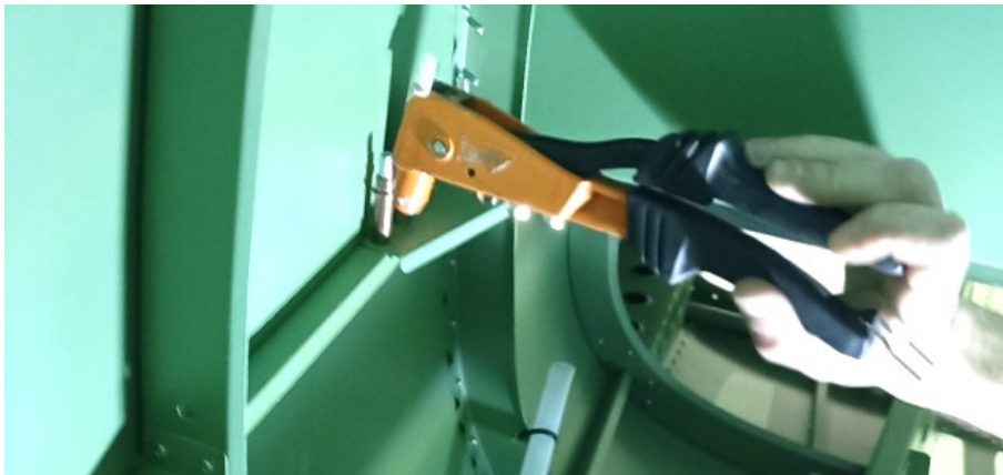
Fig. 10 Install the rivet. Repeat for other missing rivets between the clecos.
